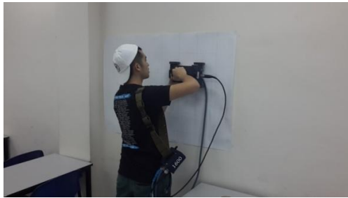
Figure 5: GPR Scanning On Area 3 (Wall)
