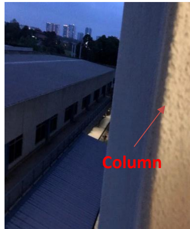
Figure 10: Column Behind the Wall
