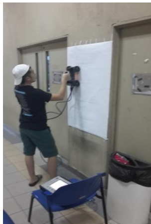
Figure 7: GPR Scanning On Area 5 (Column)
