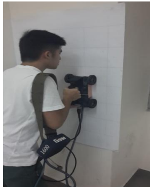
Figure 6: GPR Scanning On Area 4 (Column)
