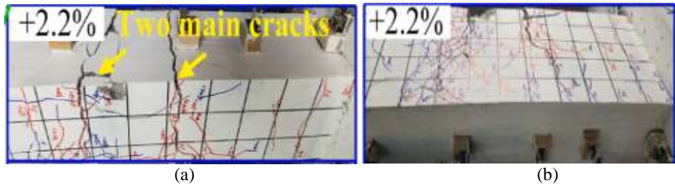
Figure 10: Cracking Formation of Experimental Beam RCB-KB5 by Qiang et al. (2019) (A) Top View of the Beam (B) Bottom View of the Beam
