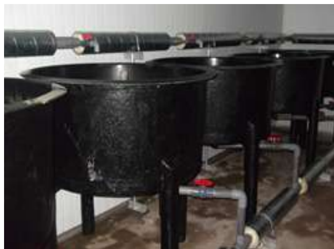
Ten fibre glass tanks in cold room with capacity of 300 L each
