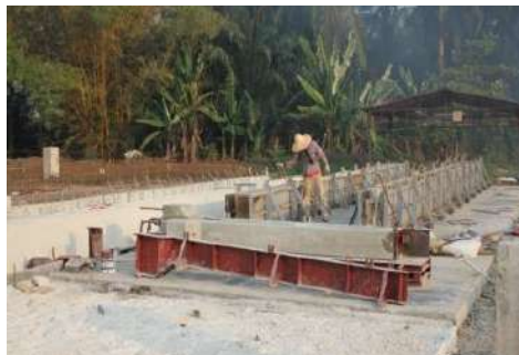
Column ready to be installed
