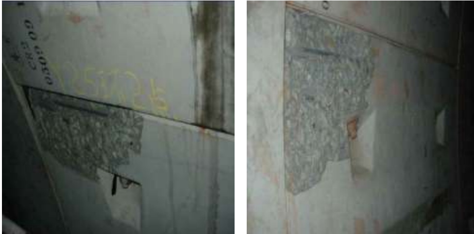
Figure 1: Damage to ordinary reinforced concrete shield segment
